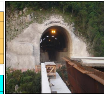
Figure 1 -Imb. North Tanagro tunnel and portal on Tanagro bridge
