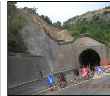
Figure 2 -Imb. South enlargement of Castelluccio tunnel
