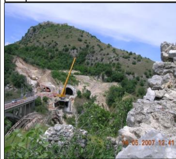
Figure 4 - Castelluccio Tunnel - Petroso arch-bridge and V. Costa Incoronata
