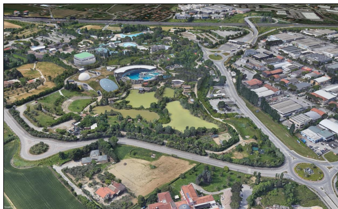
Aerial view of completed infrastructure
