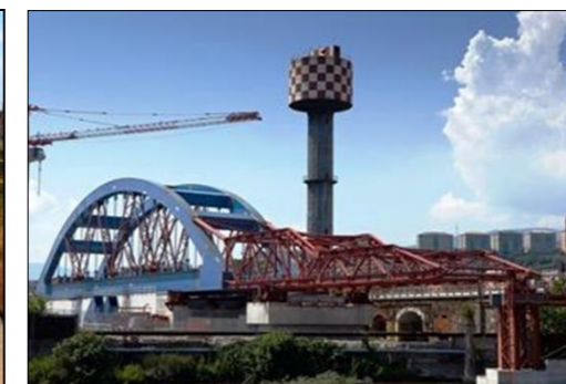
Foto 1 – Bridge launch of first span of the Polcevera bridge
